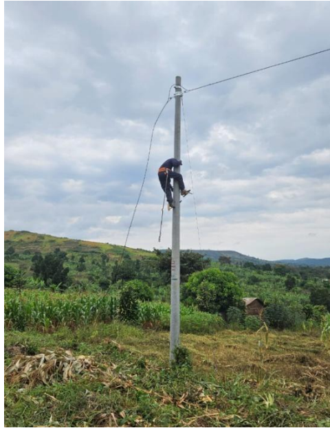
Figure 2.3—3: Technician deploying Government of Uganda fiber in Kiboga District, under NITA-U project)
